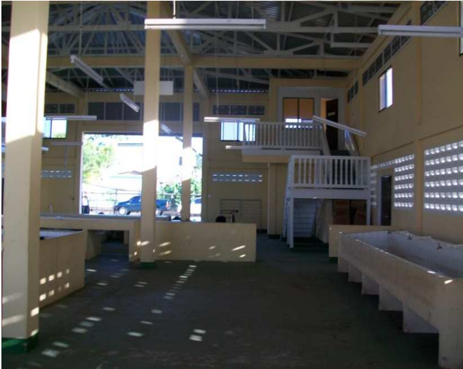
Figure 7.2(a): Internal view of the Parika Packaging Facility
